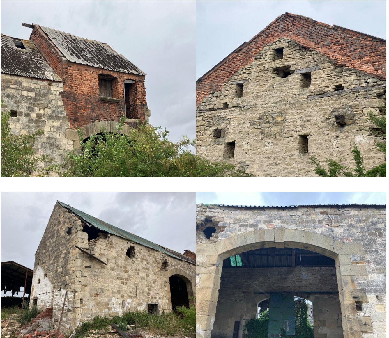
Photograph 5-8: Structure B2 (Internal and External)
